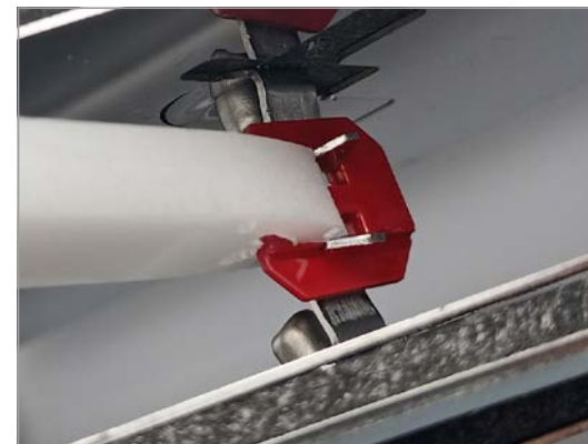
Attach/hang the fuse link to the fuse link holders of the two damper blades using the assembly tool.
