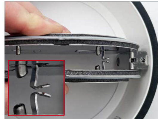
Move the damper blades from the "Closed" safety position to the "Open" position.
